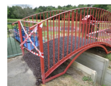
New Bridge Surface
